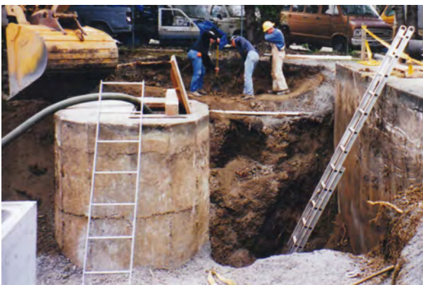
Manhole in Excavation
