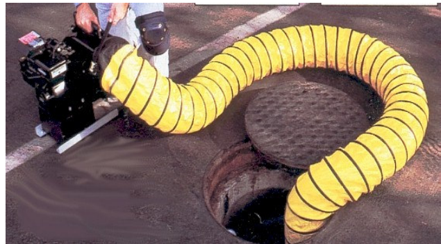
Ventilation must be continuous when there is an existing or potential atmospheric hazard.
