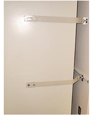
Freezer tethered to wall-anchoring system
